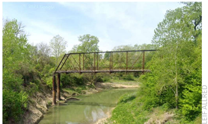
Sparks Bridge spanning Little River
