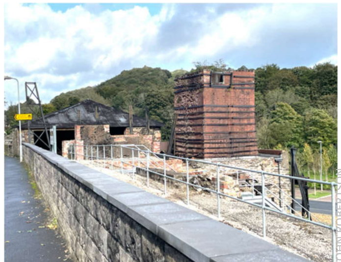
Old Ironworks Blast Furnace Relics
