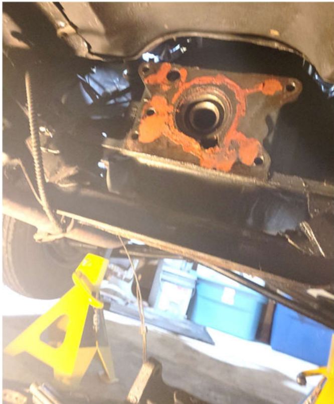
If it's not leaking, it may be empty . . . or it could be sealed shut with silicone
